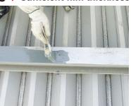
Total dry film thickness = more than 80µm Do not spread the paint too thin.
