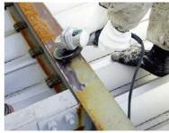
Prepare the metal surface by sandblasting or with appropriate power tools.
