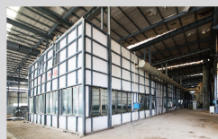
Enclosed Pickling House
